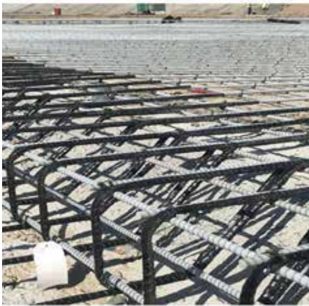
ARAMCO Jizan Flood Channel, KSA
